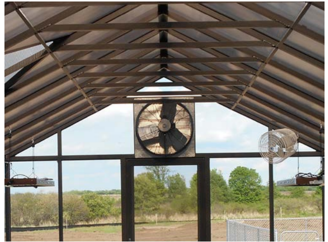
Shutter fan and circulating fans work together to quickly exchange air and maintain even temperatures
