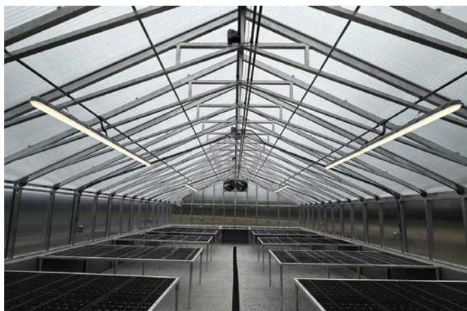
Welded Truss Engineering
