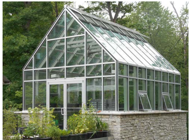
Ridge vents, side vents and windows create natural, efficient airflow for consistent temperatures
